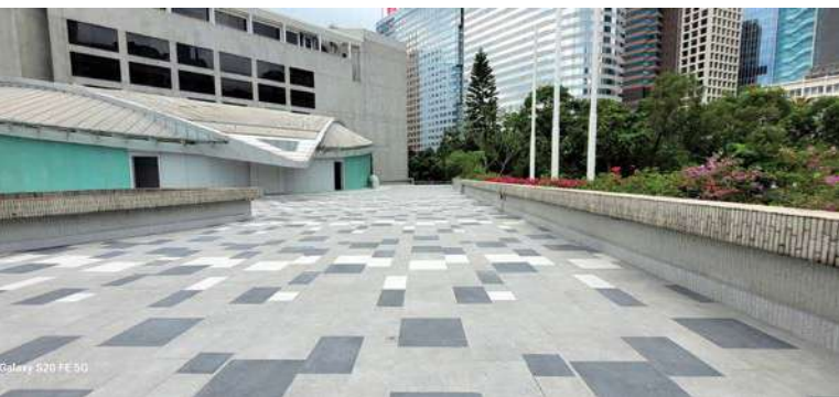
Administration Block re-roofing work. 行政大樓天面防水工程。
